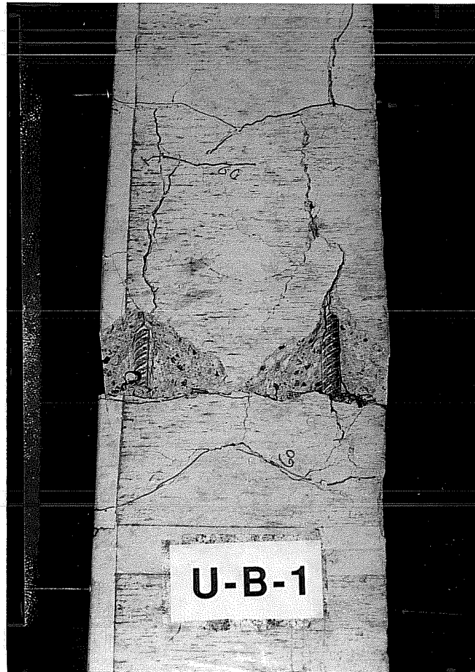
Figure 35. Failure mode of U-B-1.
